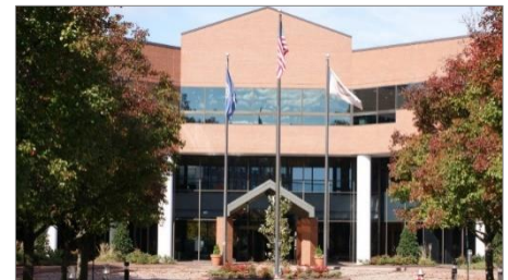
The future home of the IAFC is located in Chantilly, Virginia, about five miles west of the current Fairfax location.
