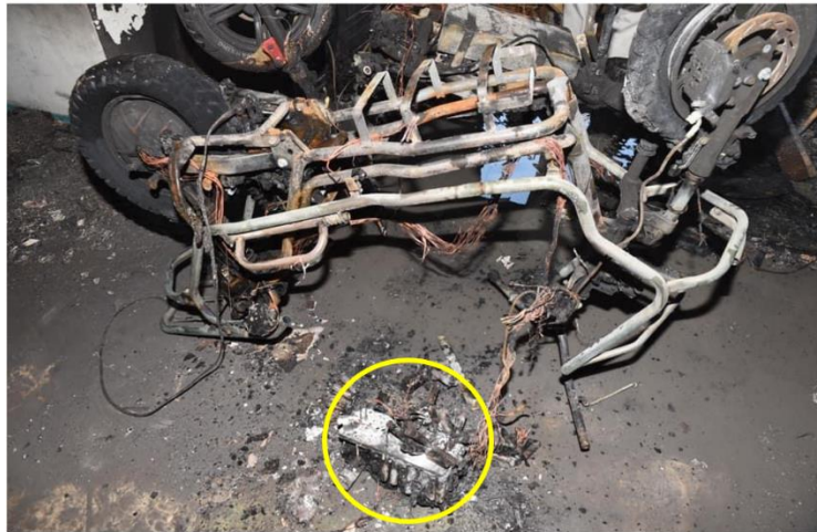
At Bronx Box 2867 (1/12/2021) a lithium-ion battery powering an e-bike sparked a blaze. Several civilians & a firefighter were injured. (Battery circled above).
