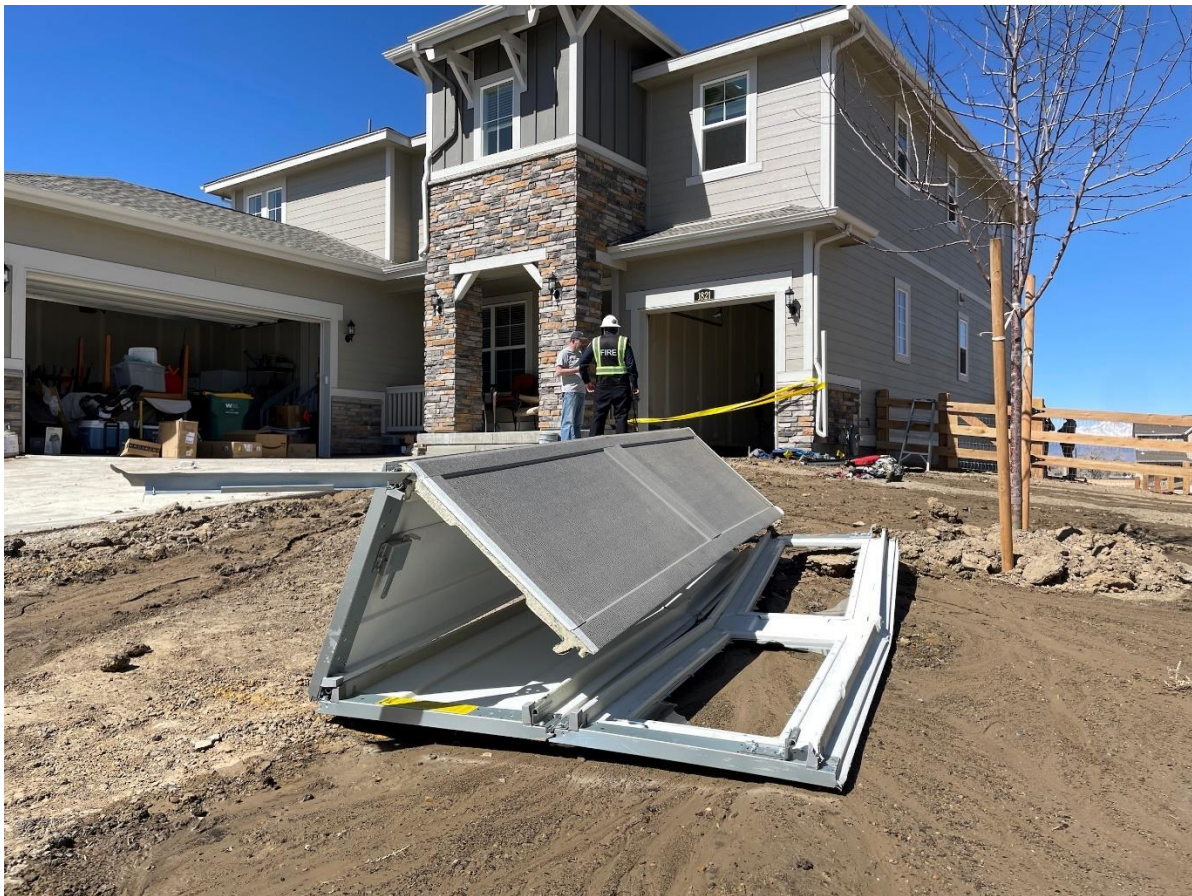
Figure 21 – Garage door location following garage explosion [26].
