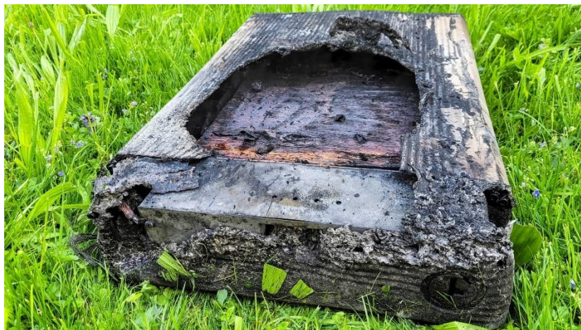
Figure 17 – Battery condition following incident [23].
