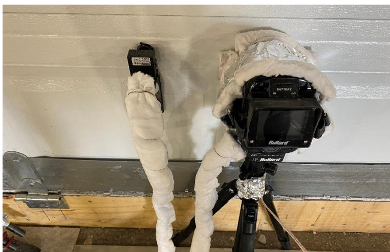
Figure 43 – HD camera (left) and TIC camera (right) installed through garage door.
