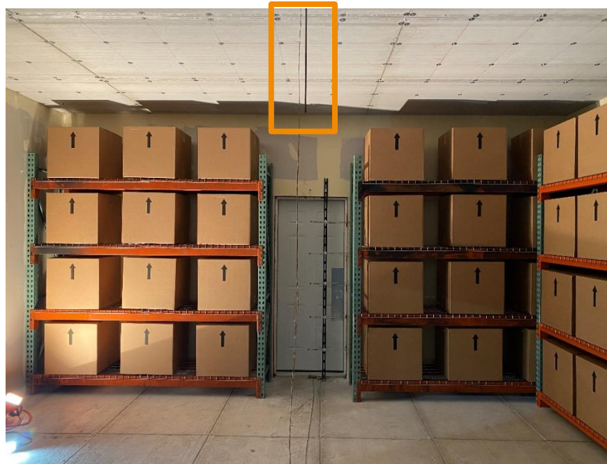
Figure 41 – Location of ceiling gas probe (outlined in orange).
