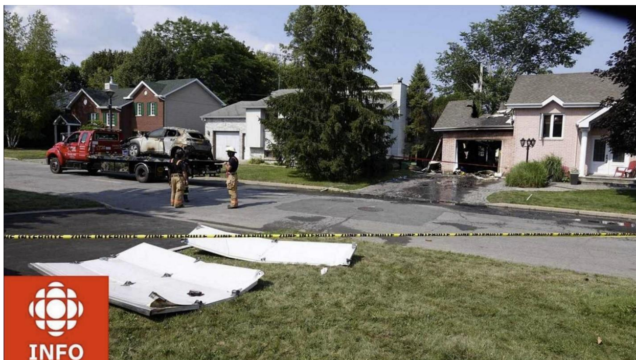
Figure 12 – Garage condition following incident [19].
