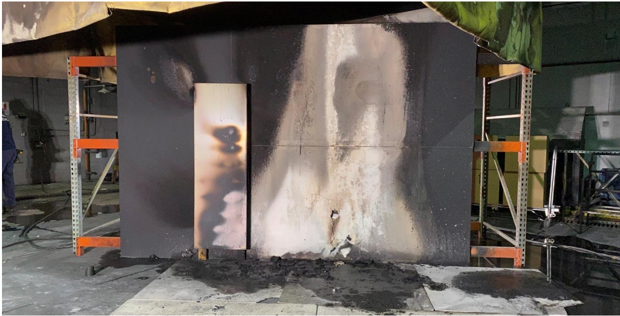
Figure 199 – Post-test condition of ESS unit and Commodity boxes in Scenario 2.
