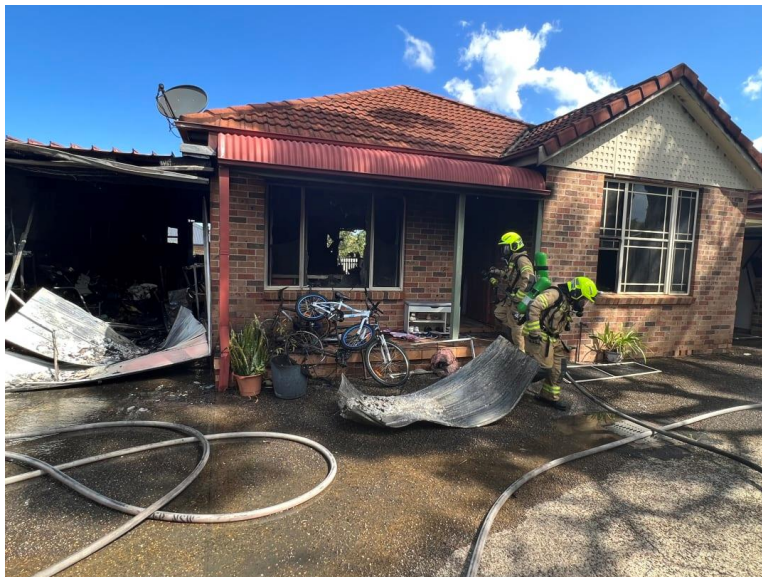
Figure 19 – Conditions after fire caused by residential ESS [25].
