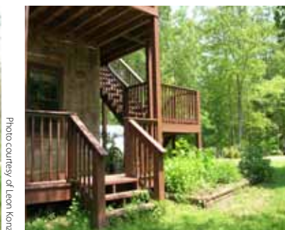
Area before and after fuel treatment. Removing this entire tree prevents a ground-level fire from reaching the deck or stairwells.
